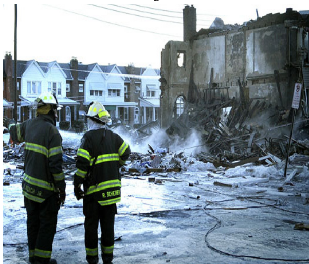
Photo Courtesy of The Morning Call Firefighters inspect the scene of the gas explosion in Allentown on N. 13th Street.
